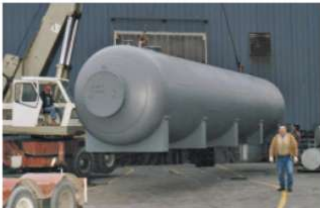
Lifting the heaviest air receiver built by Manchester.
